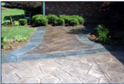
With only half of this slab sealed, it's obvious to see the color enriching benefits of a sealer. Photo courtesy of Decorative Concrete Institute .
