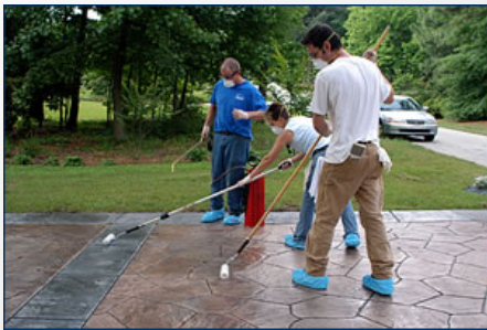
Photo Courtesy of Decorative Concrete Institute .
