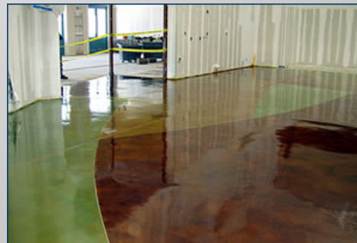
Photo courtesy of Decorative Concrete Institute .
