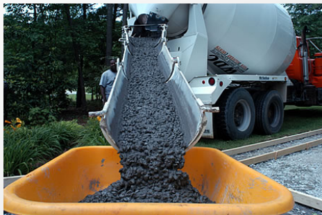
Photo courtesy of Decorative Concrete Institute .
