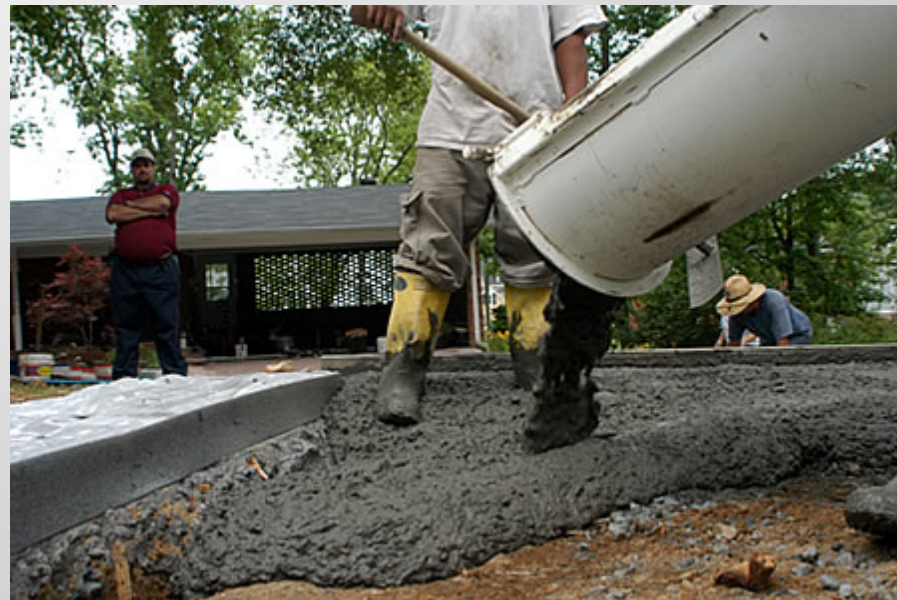
Photo Courtesy of Decorative Concrete Institute .
