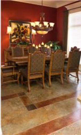
Acid-based stains produce natural color variations in the concrete. Kemiko Concrete Products in Leonard, TX.
