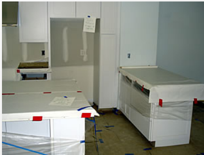
Cast in place job with curing blankets taped in place.
